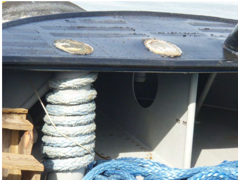
Figure 2.10 Failure of a Badly-Designed Towing Staple
