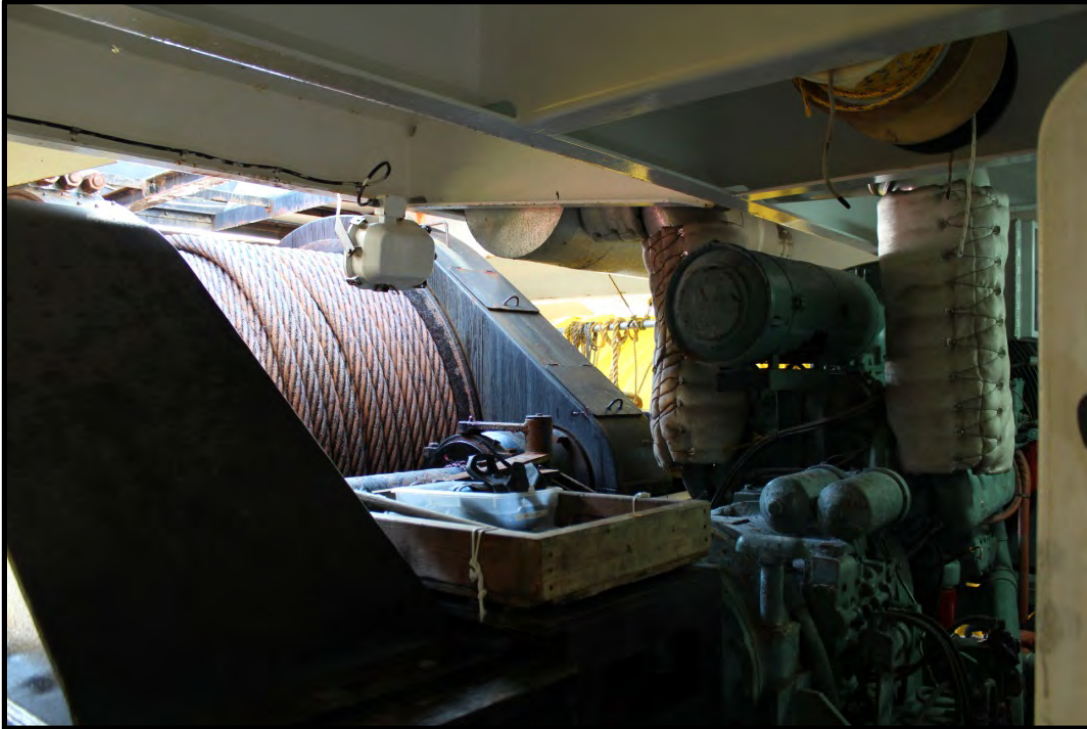
Figure D.4 - View of forward end of aft towing winch, showing the direct diesel engine drive and the wire stowage drum.
