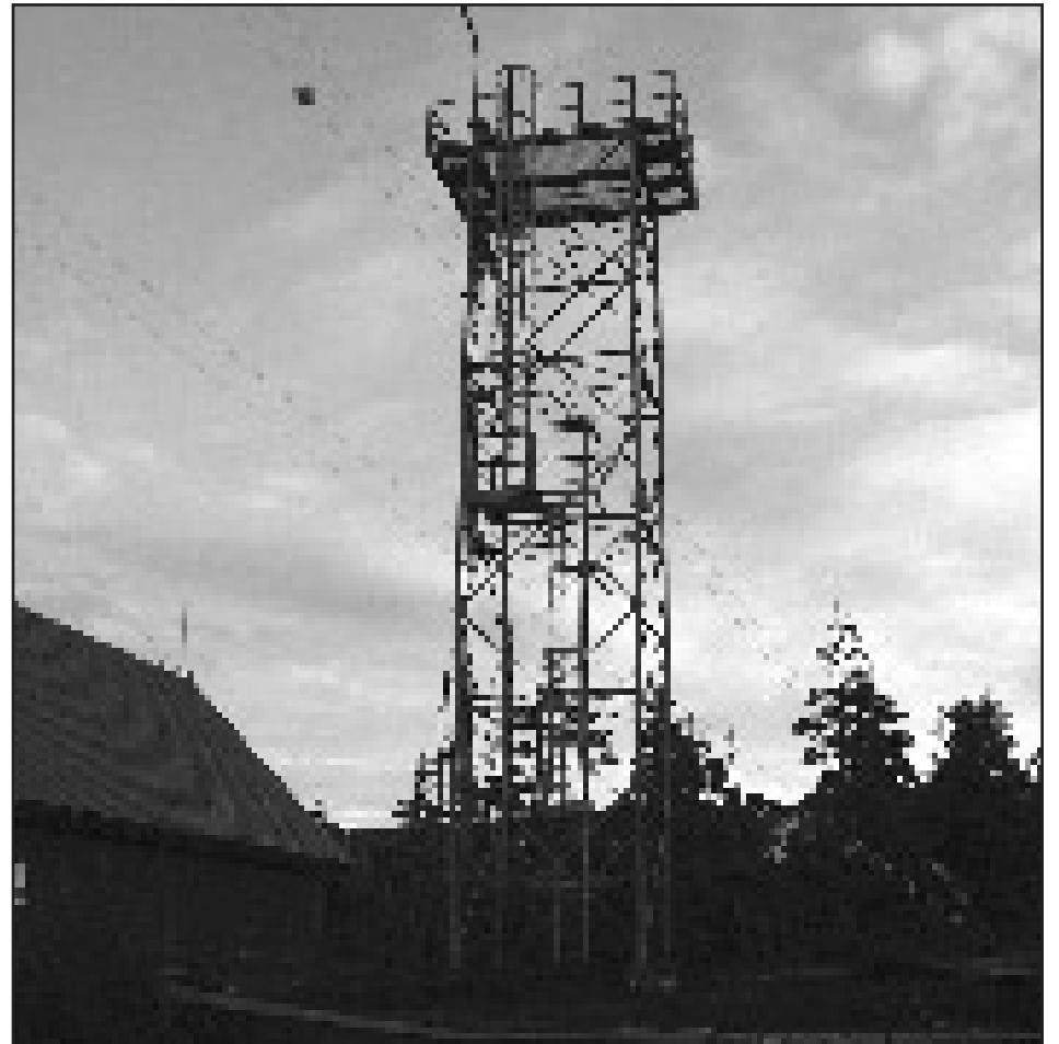
This tower on Reef Island will soon house a radar system for detecting icebergs in the tanker lanes. Photo by Rhonda Arvidson
