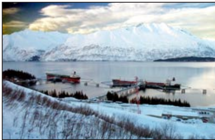
The latest contingency plan for the Valdez tanker terminal, shown here, contains several improvements sought by the citizens' council. Photo by Tom Kuckertz, citizens' council.
