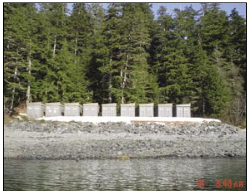
STILL SNOWED IN: A month later, on April 16, the berms were still present, though reduced in size by warm spring weather. The council has called for an independent entity to verify that response depots like Main Bay are regularly inspected and properly maintained. Photo source confidential.
