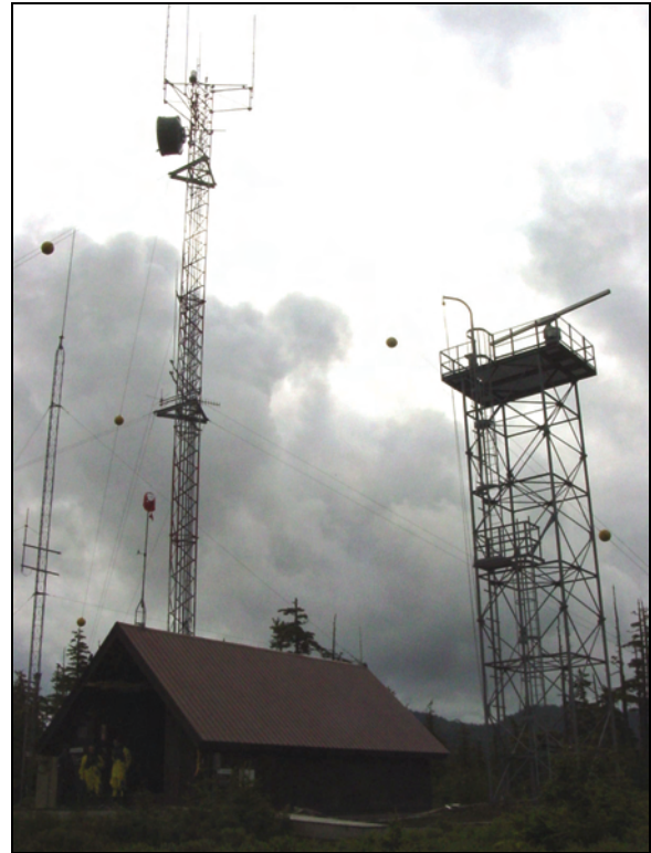
Figure 2-1. Reef Island radar site showing SERVS equipment shelter, microwave communications tower (left) and radar tower (right)
