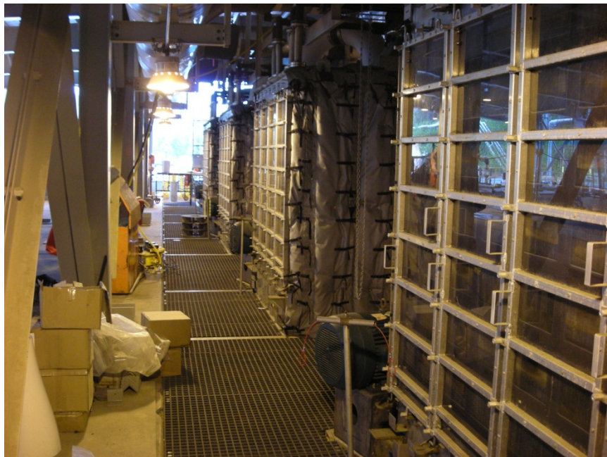
Seven-tray air stripper units at the reconfigured VMT BWTF (photo: J.A. Kalmar)
