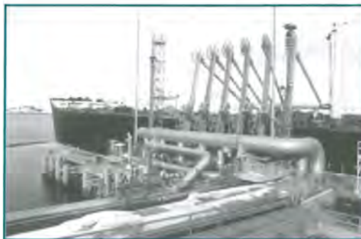
New equipment at Berths 4 and 5 collects oil vapors from tankers during crude oil loading.
