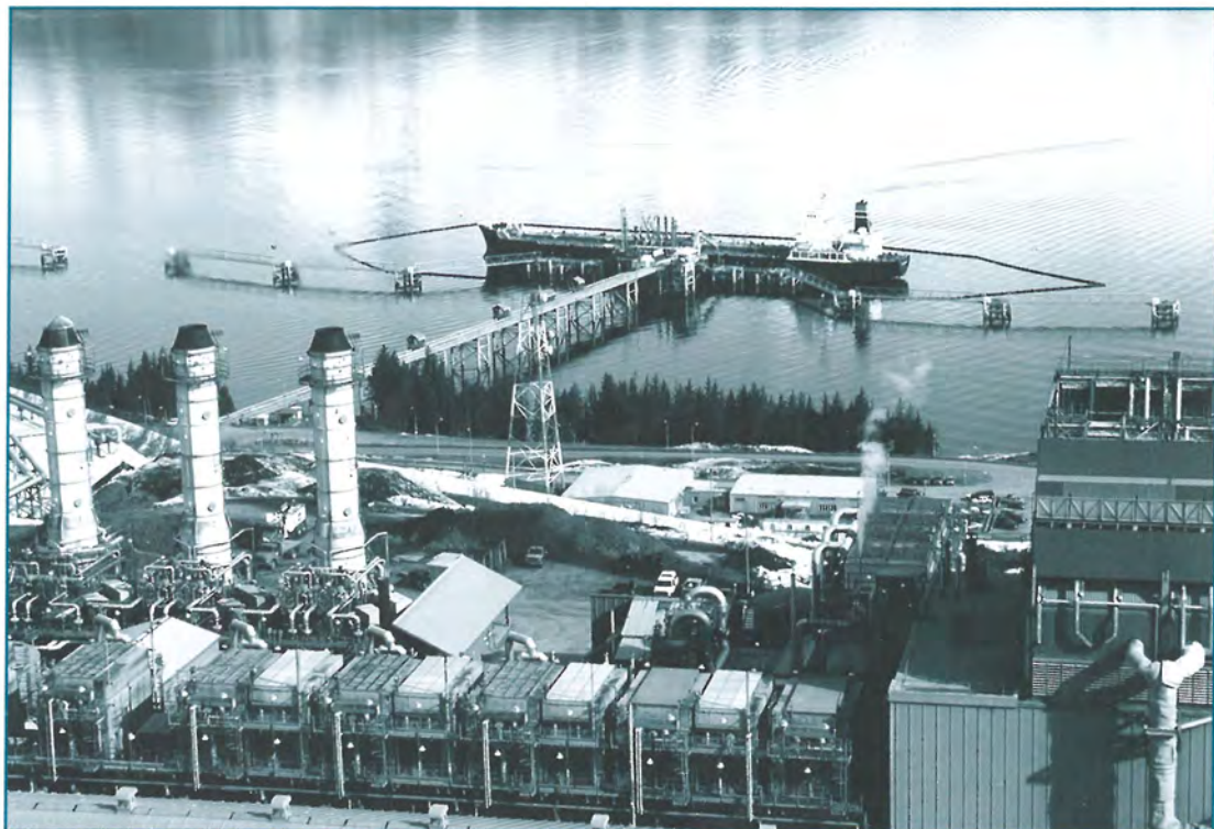
The SeaRiver Puget Sound takes on oil at Alyeska's Valdez terminal. The three chimneys at the left side of the picture are the incinerators that burn oily vapors forced out of tanker cargo holds during loading.
