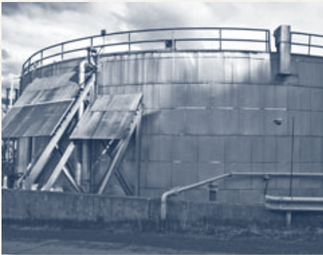
This storage tank is part of Alyeska's facility for treating oily ballast water that comes off of arriving tankers. Photo by Tom Kuckertz.
