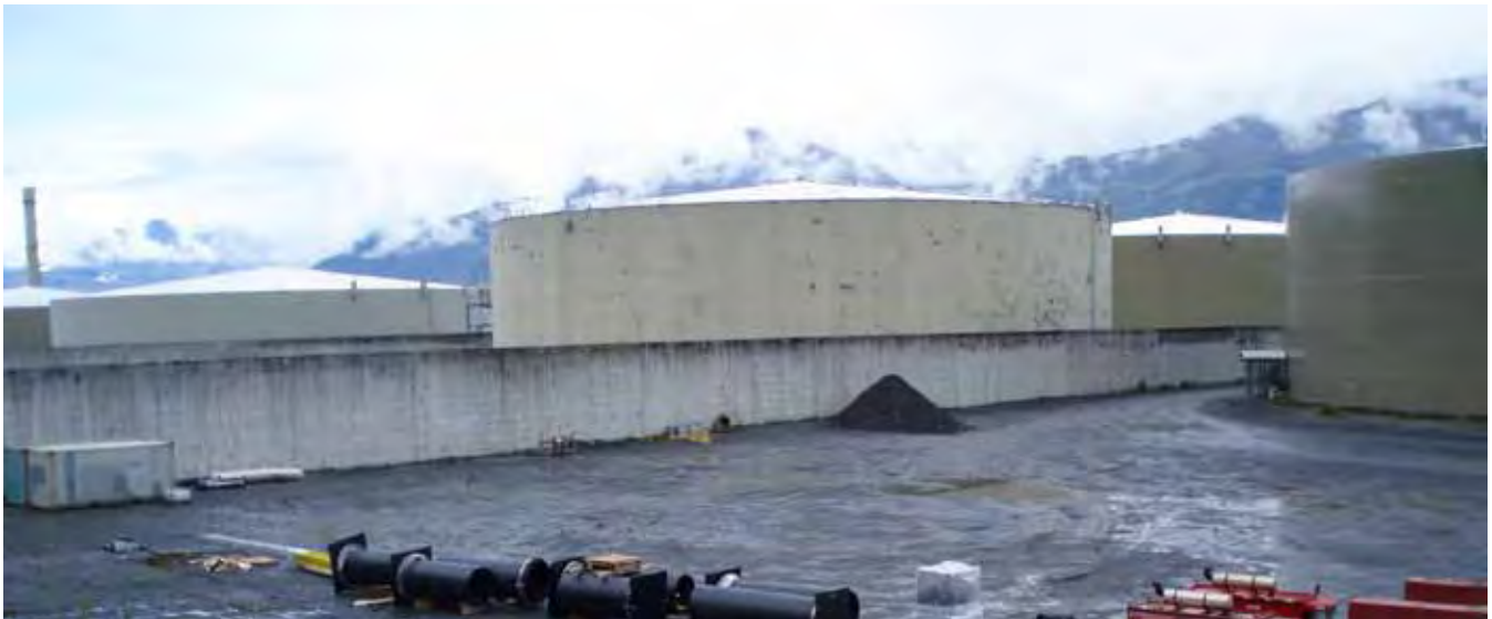
These giant tanks at the Alyeska terminal in Valdez are used for storing arriving North Slope crude until it can be loaded onto tankers for shipment south. Photo by Tom Kuckertz.
