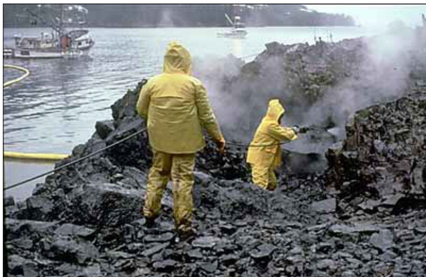
Workers used high-pressure, hot-water washing to clean an oiled shoreline in Prince William Sound after the 1989 Exxon Valdez oil spill. (NOAA photo)
