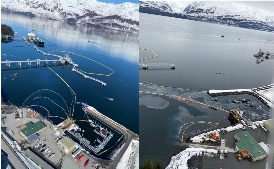
Fig. 2. Spill site and visible oil and sheen observed inside the containment booms at Valdez Terminal in April 2020. Photos courtesy of Alyeska Pipeline.
