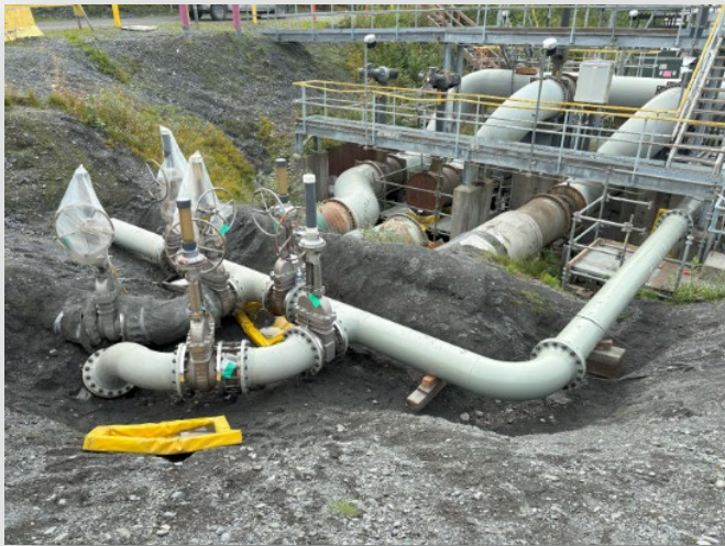
Ballast Water Treatment B Header Inspection
