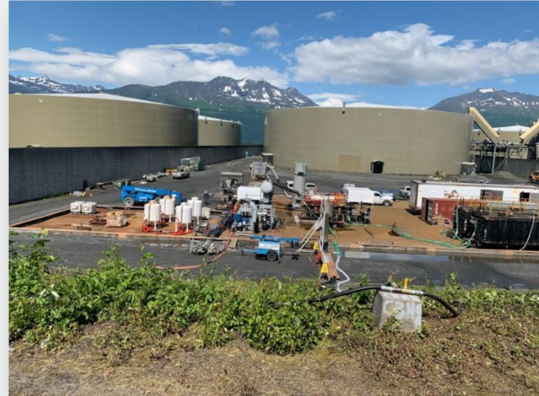
Tank 5 API Inspection and ILI of Crude Oil Branch Lines
