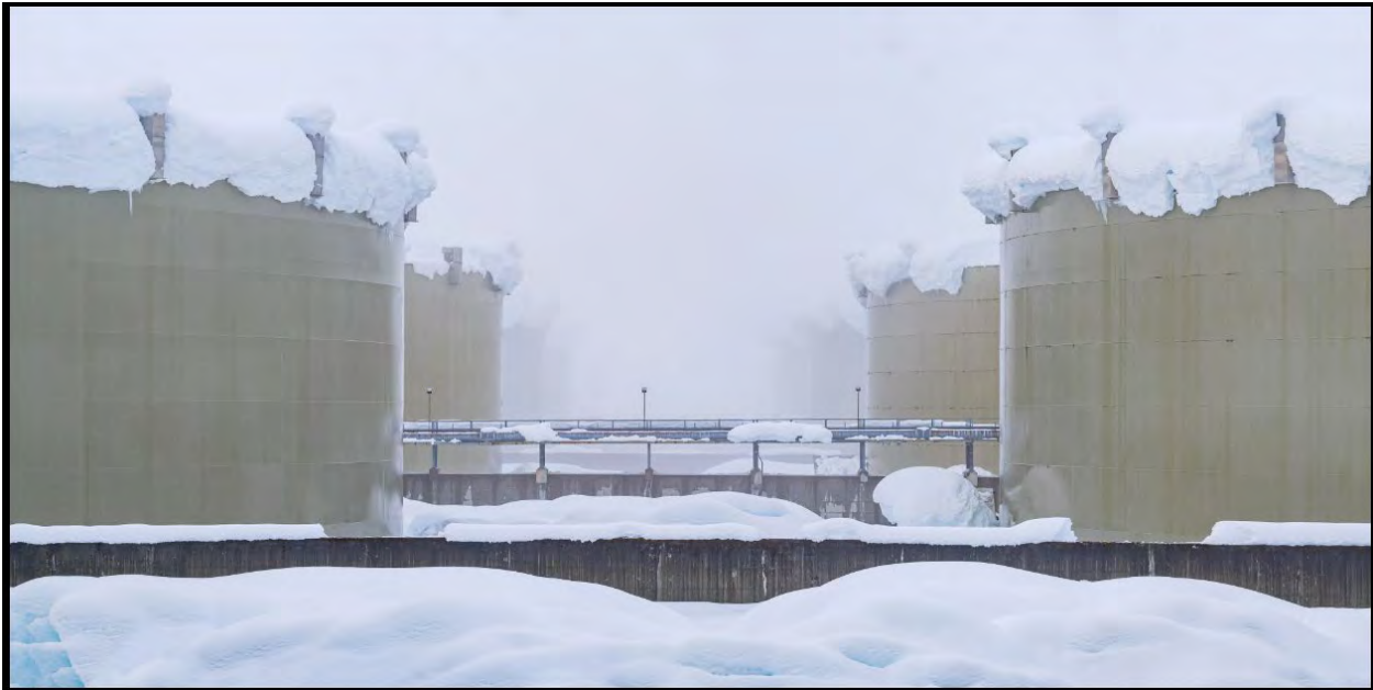
Figures 6A through 6G – Examples of Snow Loading and Damaged Tank Vents
