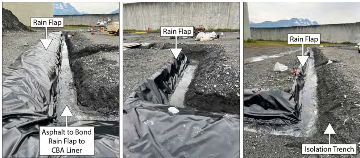
Figure 3. Photographs of installed rain flap (from WSP 2024a).
