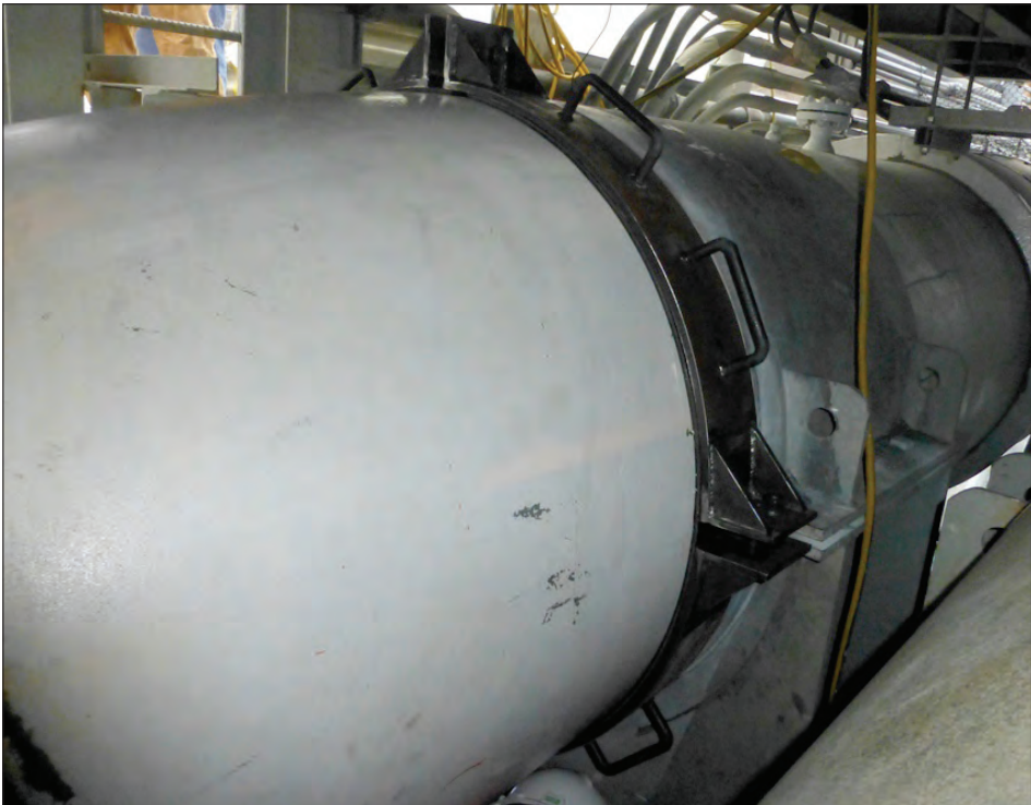
A temporary black carbon steel clamp was installed to prevent an oil leak from the localized corroded area. Photo courtesy of Alyeska.
