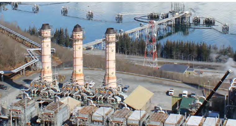
Vapors from crude oil are captured and converted into energy that helps power the terminal.
