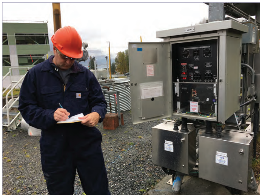
Left: Keith Boswell from National Pipeline Services observes cathodic protection system equipment at the Valdez Marine Terminal in 2019. Photo by Diana Bouchard.
