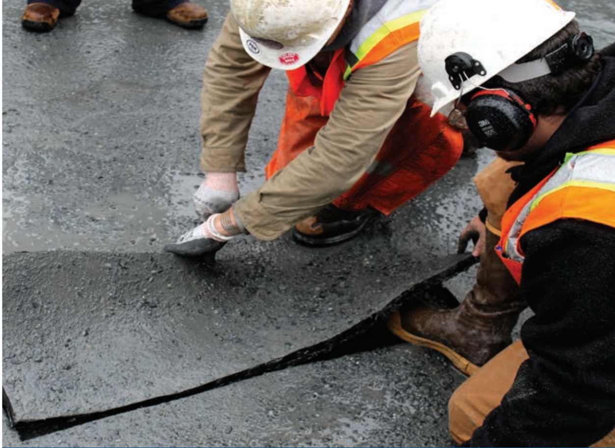
The secondary containment system surrounding the tanks includes an asphalt liner, buried under several feet of gravel and dirt. From 2014-2017, Alyeska dug up a section of the liner to test for damage.
