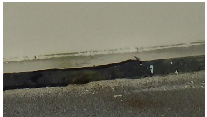
Figure 9 – Annular Plate Extension (Sealed)
