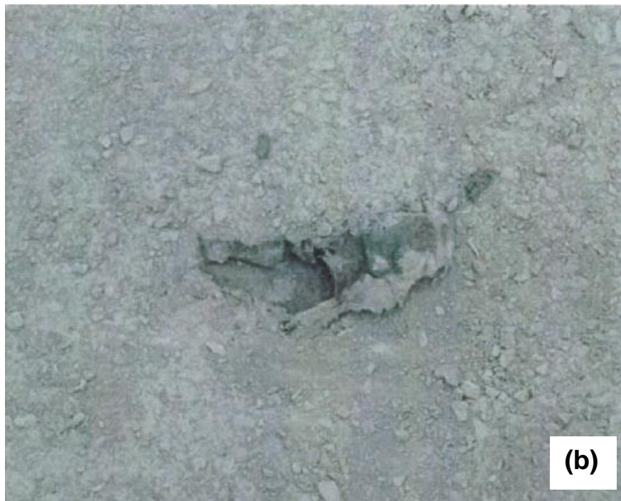
Fig. 2.1. Removing overlying gravelly material from the VMT secondary containment area to expose the CBA liner (a). Defect encountered during visual inspection of the liner (b) (from Golder 2015).
