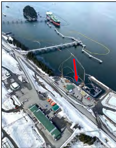
Figure 1. Containment booms placed around the spill site (red arrow) and in adjacent waters at the Valdez Marine Terminal. Saw Island is in the background upper left, adjacent to a Berth 5 tanker. Image from Alyeska Pipeline Service Company.
