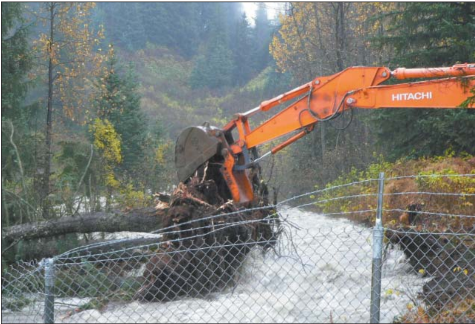
BELOW: Alyeska maintenance personnel and contractors removed multiple trees as they fell into Allison Creek. The trees’ weight threatened to destroy a bridge, but removing them helped save the structure.
