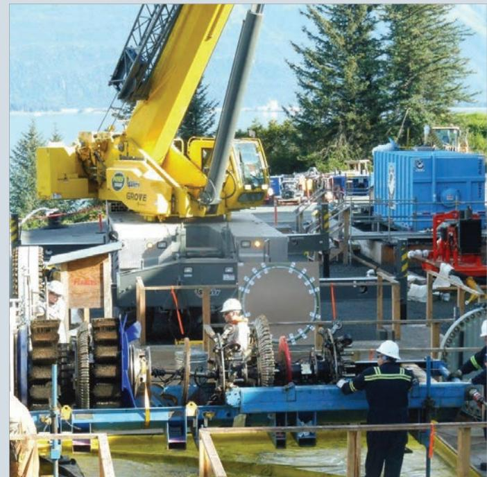
Crews insert an In-Line Inspection tool B header on the Valdez Marine Terminal.
