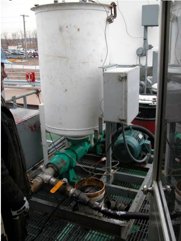
Figure 4 The Hopper Tank and Pump Used to Deliver Oil to the Discharge Outlet
