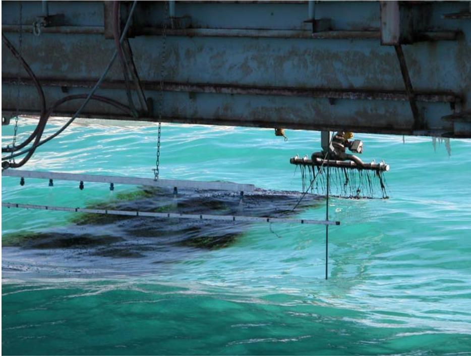
Figure 3 The Discharge Outlet. The Oil Typically Spread from 4 Feet to About 6 Feet
