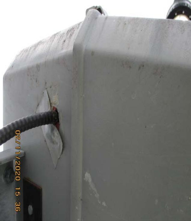
*Duct Tape is used to seal this off from a Class 1 Division 2 classified area instead of a proper sealant. AKOSH Inspection Report 1449721.015.*
