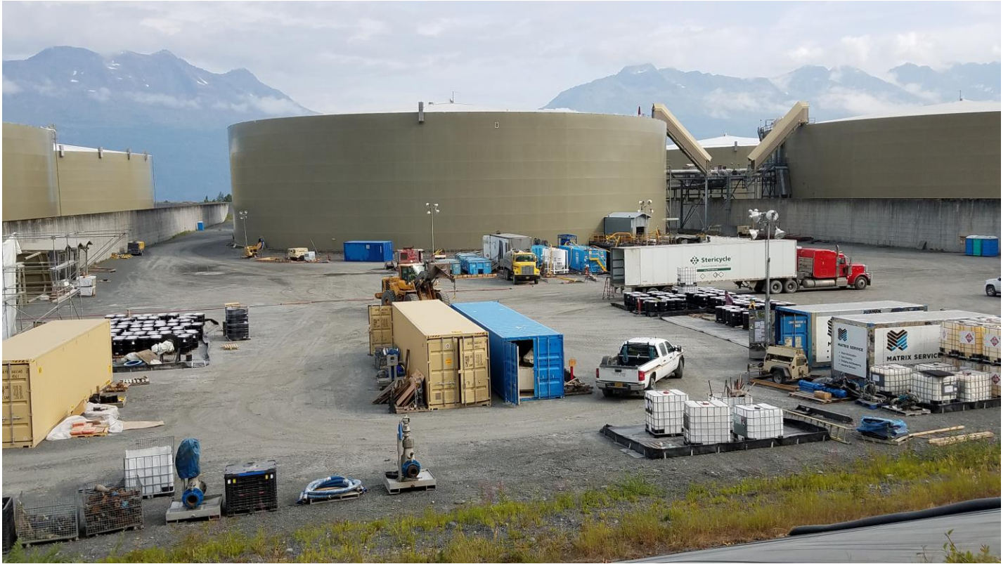
Figure 3 - Tank 8 During 2019 Out-of-Service Inspection (photo courtesy of Austin Love)
