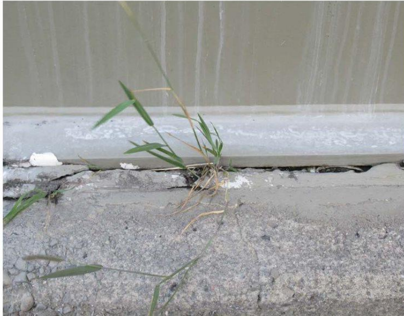
Figure 10 - Tank 8 Ringwall/Annular Plate Seal
