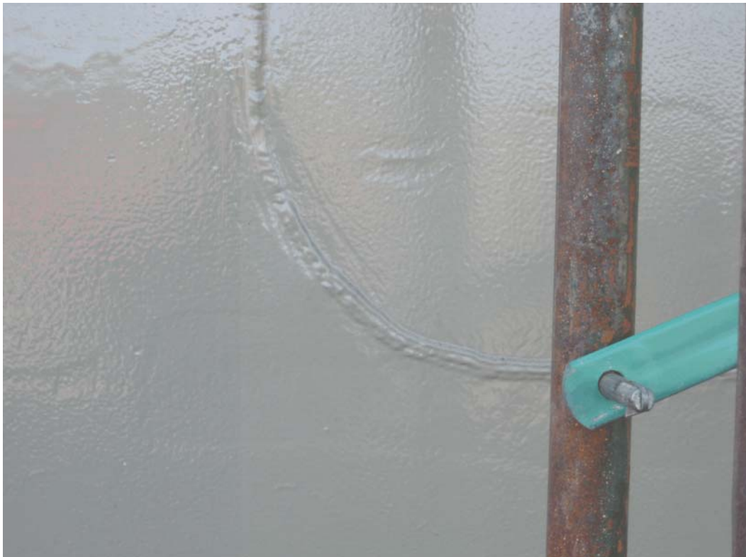
figure 6 - Close-up of a doorsheet corner weld.
