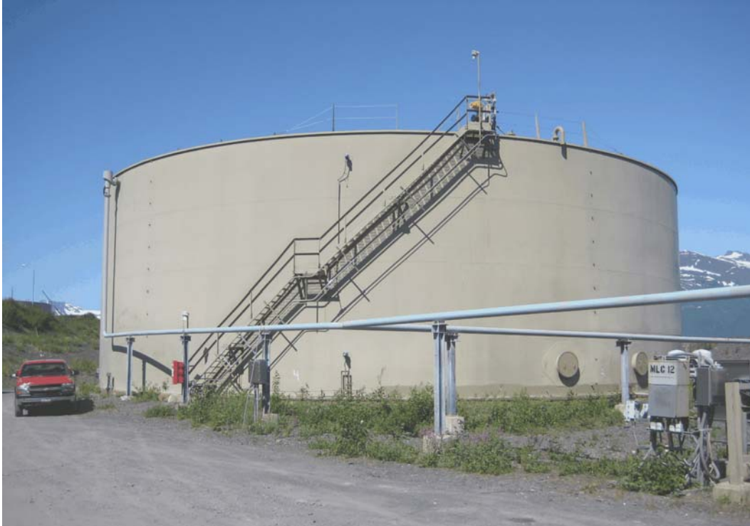
figure 1 - Tank 58-TK-55 at the APSC facility in Valdez, AK
