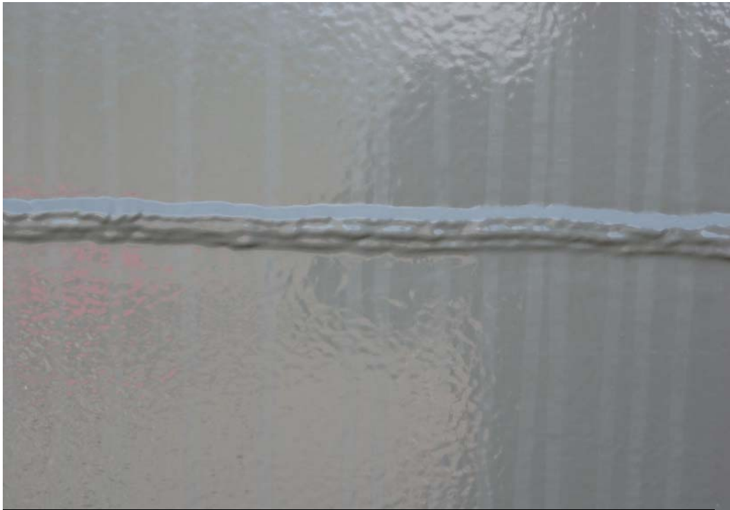
figure 8 - Close-up of a doorsheet weld, possibly representing a repair weld.
