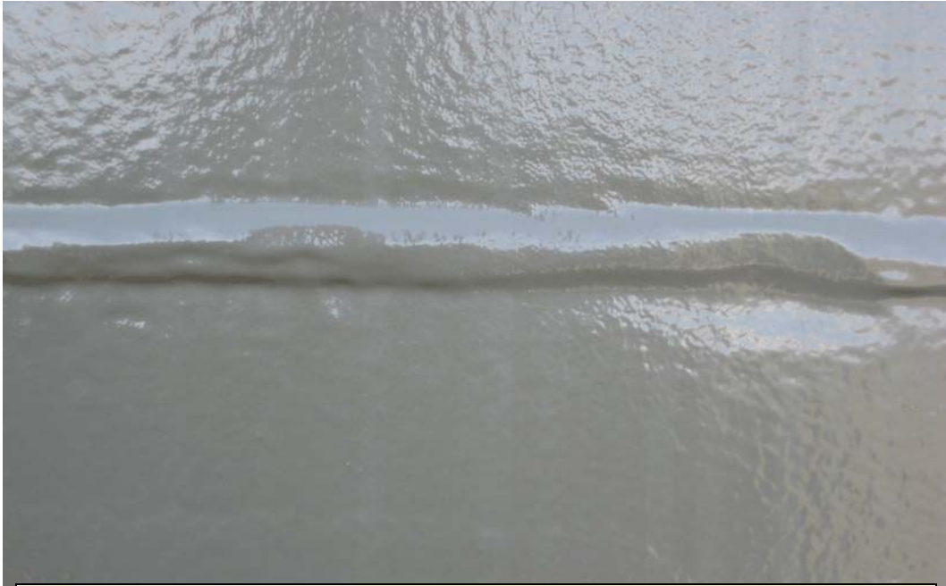
figure 7 - Close-up of a doorsheet horizontal weld.
