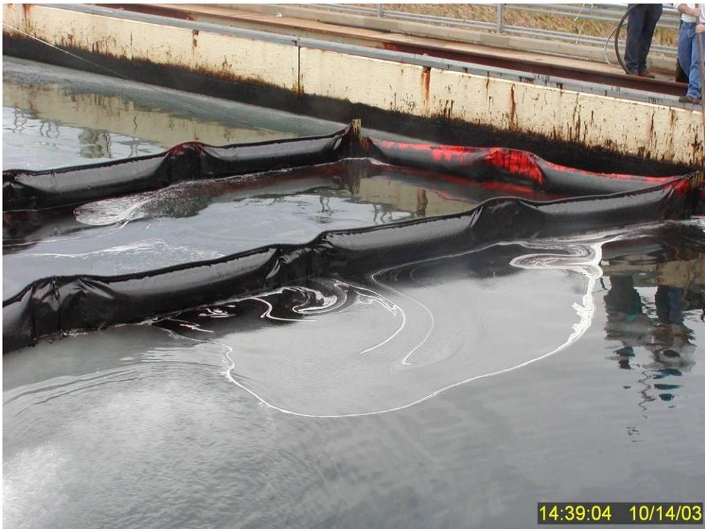
**Figure 120** Residual nondispersed oil within the primary containment boom being herded in preparation for vacuum recovery.
