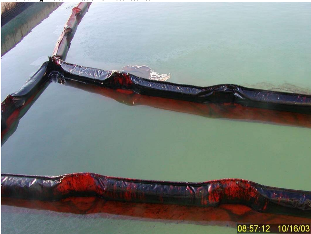
Figure 240 Residual surface oil inside the northeast corner of the primary containment boom after reestablishing the boom configuration on 16 October 2003.
