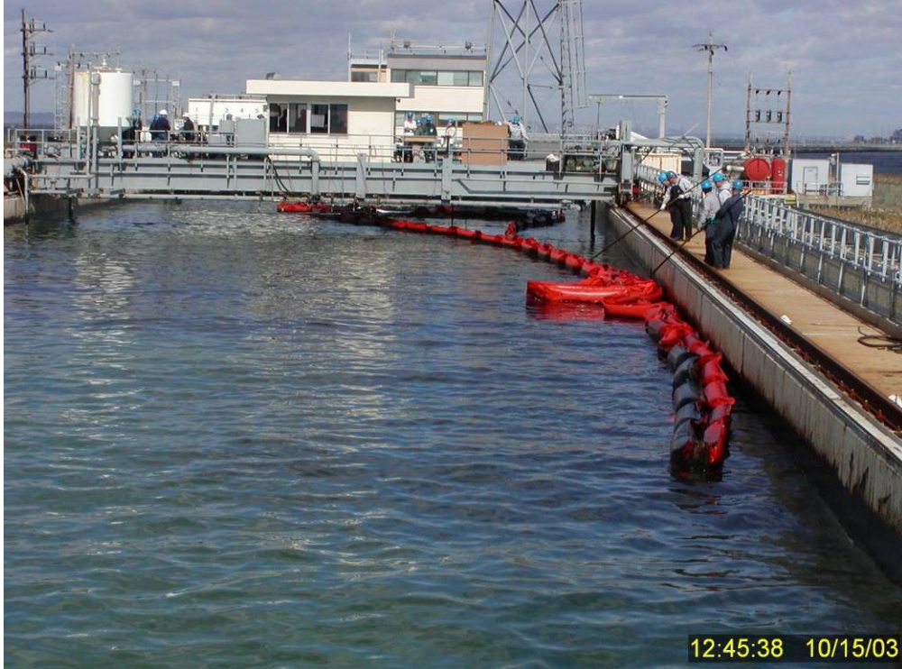
Figure 226 Initial efforts to reopen the containment boom to see if nondispersed surface oil could possibly be recovered. I have no doubt that some unknown amount of nondispersed surface oil was lost during these operations.
