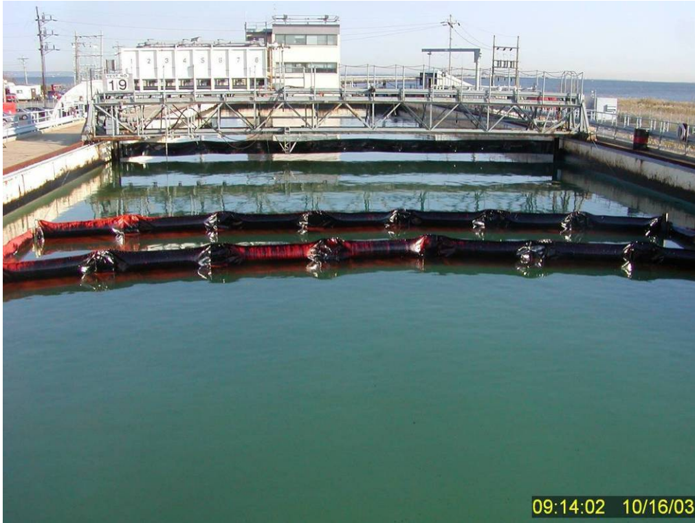
Figure 242 Permanent boom curtain beneath the northern-most bridge in raised position to facilitate tank cleaning (fire monitor herding of surface oil) outside of the test area in preparation for Test No. 19.
