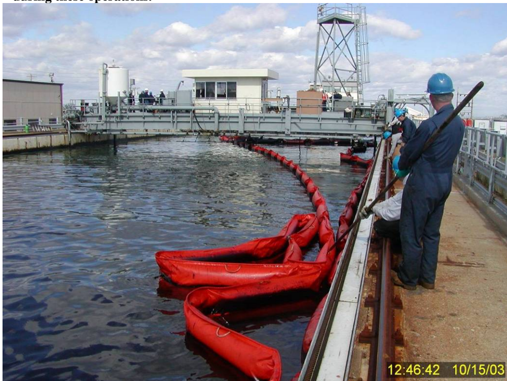
Figure 227 Reopening the containment boom for possible nondispersed surface oil recovery.
