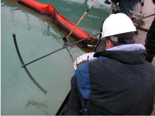
Figure 6 Recovery Operation. The Oil is Picked up Using a Cup on a Pole. Note that There is an Extensive Slick Forming on the Tank Behind the Recovery Operation
