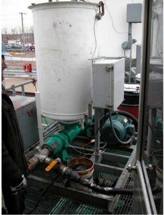
Figure 4 The Hopper Tank and Pump Used to Deliver Oil to the Discharge Outlet
