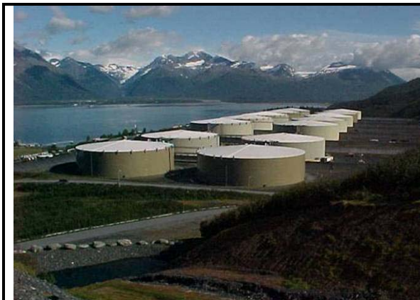
Figure 3: 510,000 barrel crude oil storage tanks
