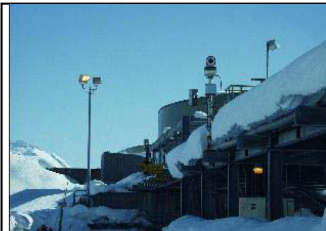
Figure 7: BWTF Storage Tank (90 series)
