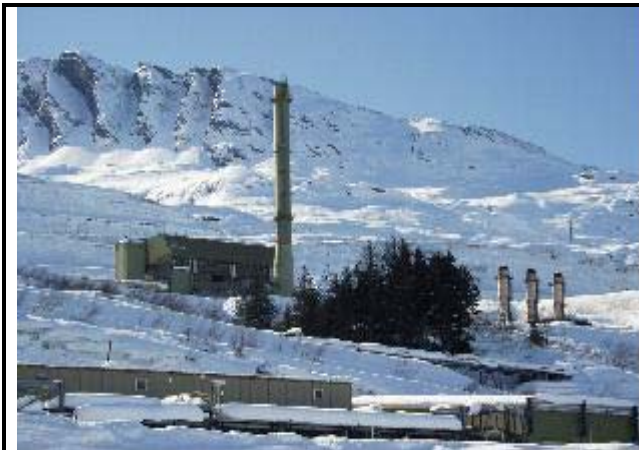
Figure 5: power boiler stack (left), three incinerator stacks (right)
